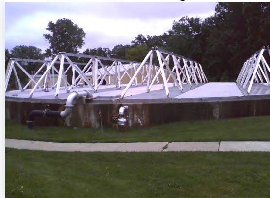
Covered Aerobic Digester
