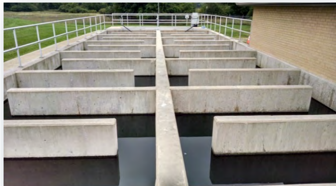
Chlorine Contact Tanks
