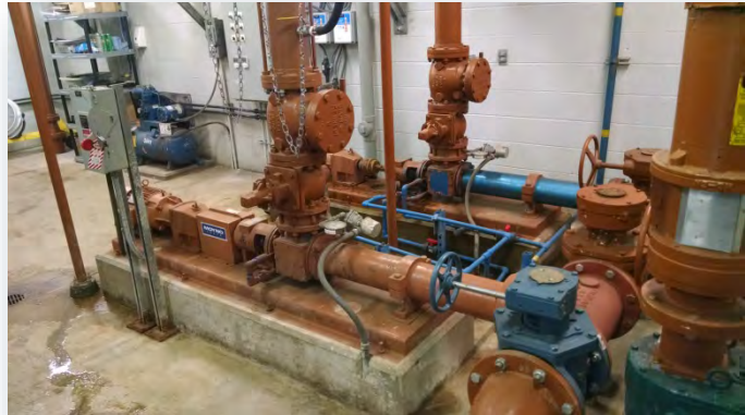
Progressing Cavity Sludge Transfer Pumps
