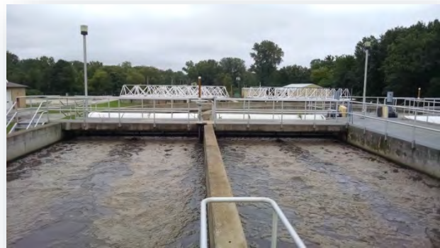
2-ring Orbal Oxidation Ditch
