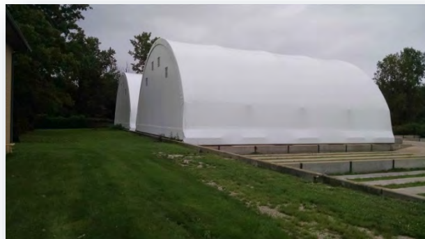
Covered Sludge Drying Beds
