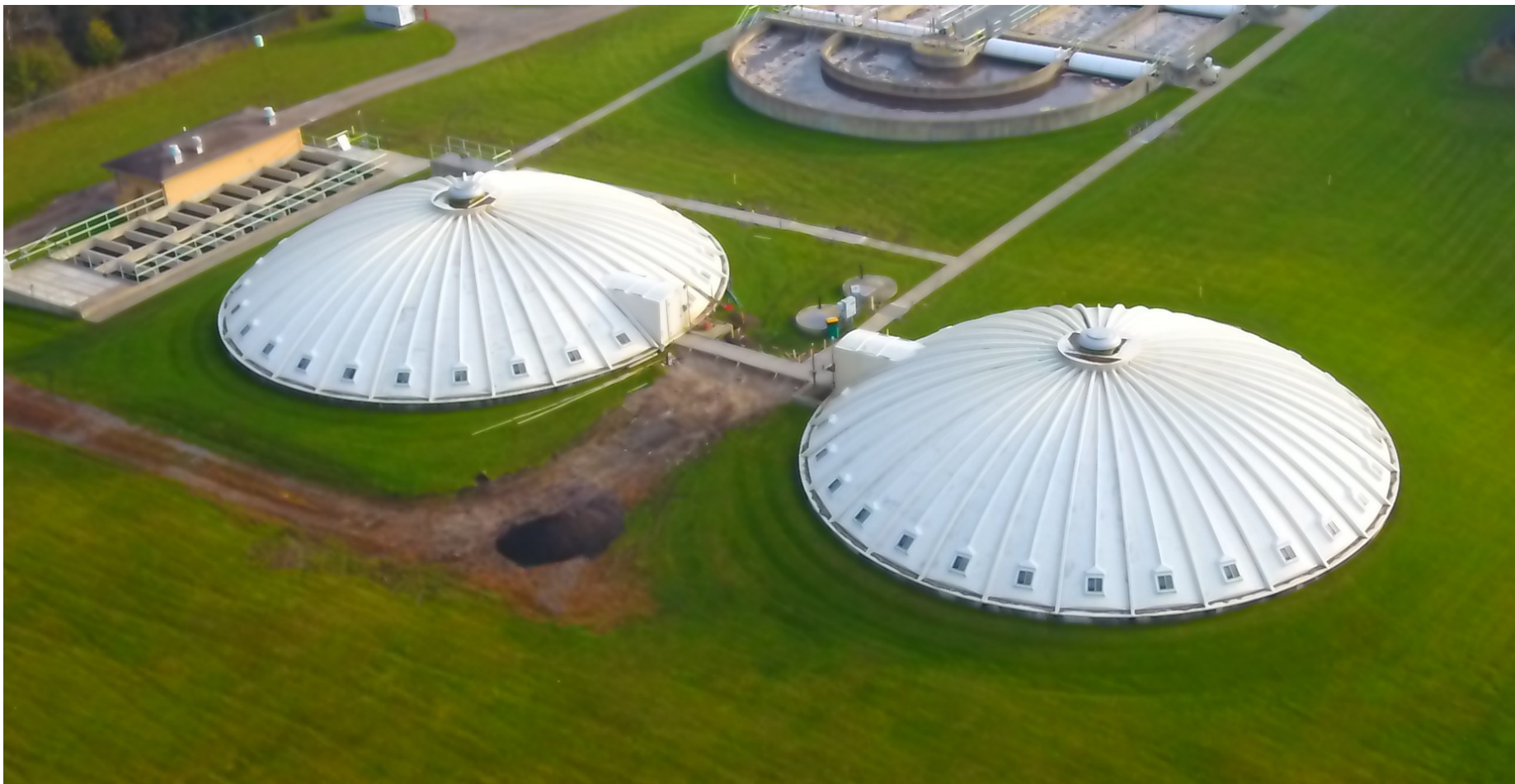
Attachment "C" – Aerial of NMWRD Secondary Clarifiers.
