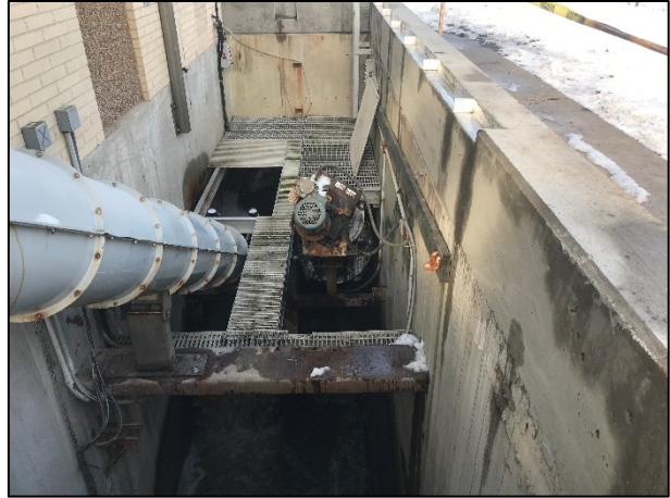
View of the removed conveyor within the wet well.
