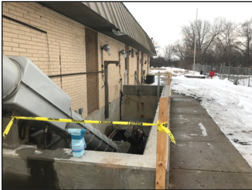
Screenings Conveyor removed from Raw Wet Well
