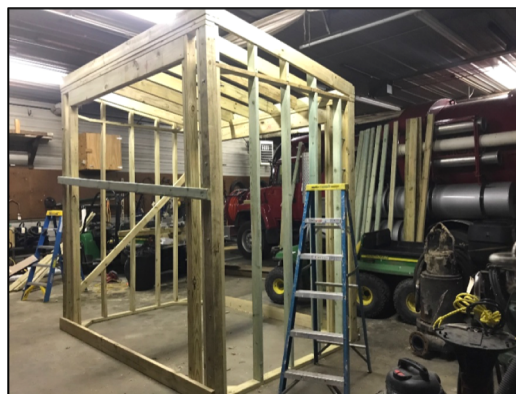
Dumpster enclosure framing
