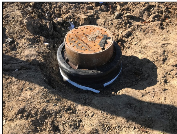
Picture of manhole after successful tie-in.
