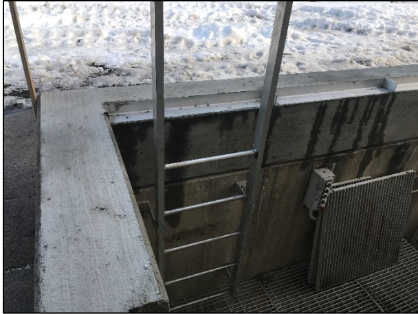
New wall mounted ladder within wet well.
