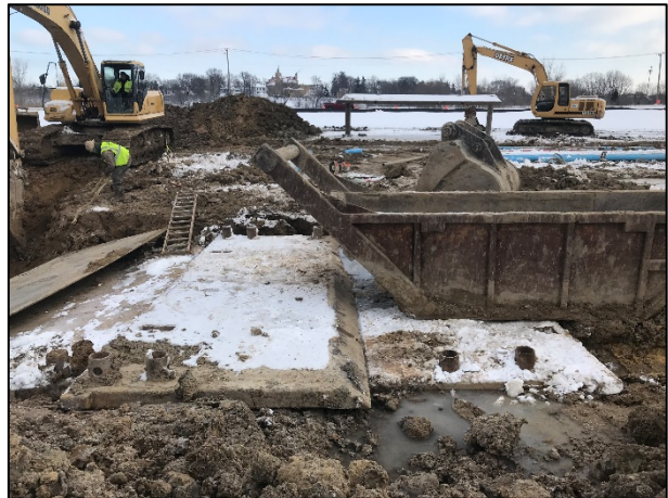
Picture of covered trench to deal with the inclement weather.
