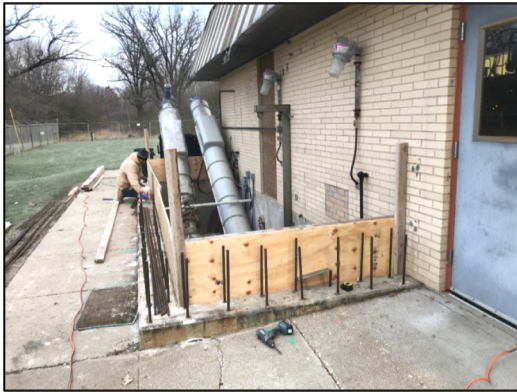
Curb form and reinforcing rebar installation
