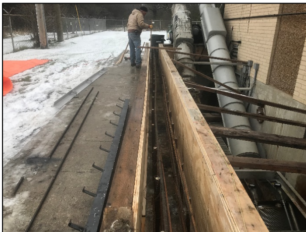
Picture of the supports that were used to pour the concrete curb.
