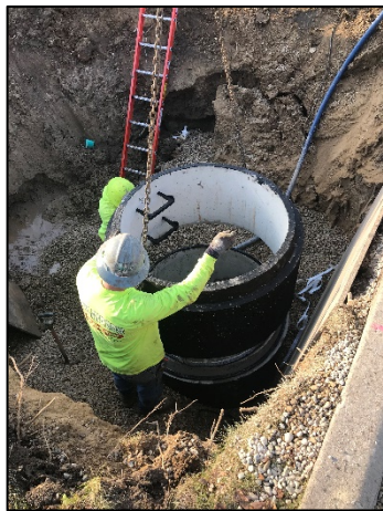
In-trench view of manhole tie-in to existing gravity main.
