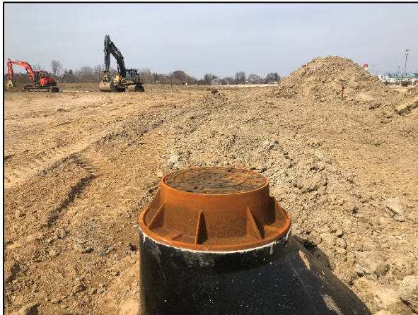
Picture of the last manhole set along Ring Road.
