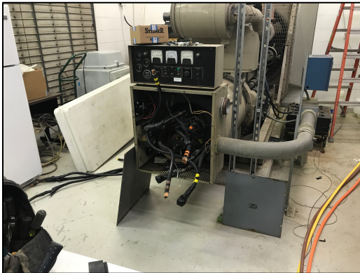
The old 1978 generator was disconnected from the plant power systems.
