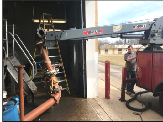
District staff removing sludge feed line from Belt Filter Press.
