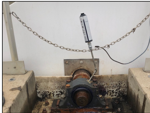
Automatic Greaser Installed on Aerator Bearing
