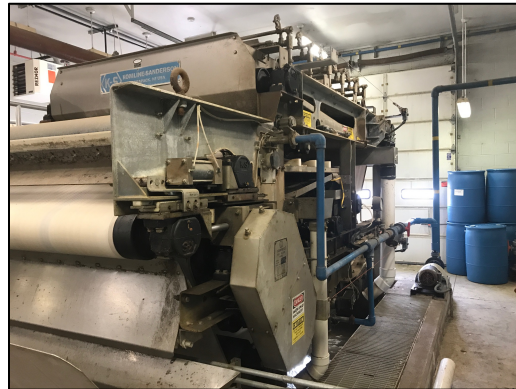
Installed in 1999, the Belt Filter Press has been replaced by the Centrifuge.
