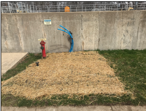
Power and data conduits for future SCADA control panel.
