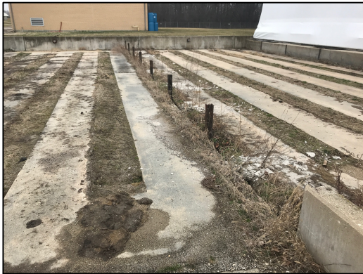
Concrete dividing wall removed with metal supports remaining.
