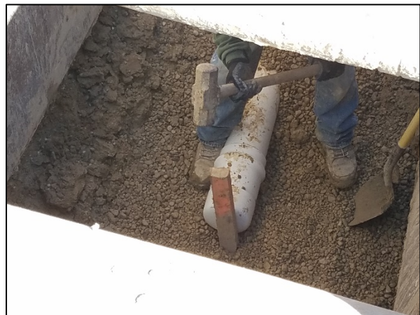
LCGC capped the service line 5 feet short of the main line.
