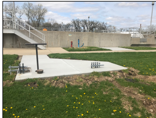
Concrete poured at control panel & valve actuator site.
