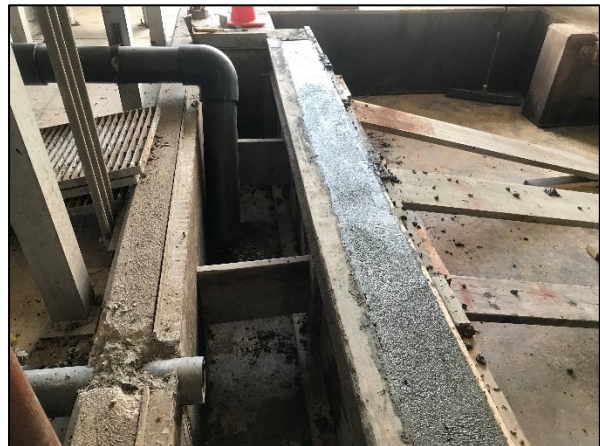
Picture of the newly poured concrete wall in the old BFP pit.
