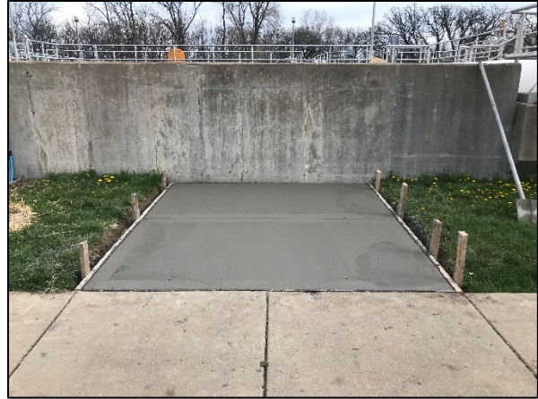
Second pad after concrete was poured.
