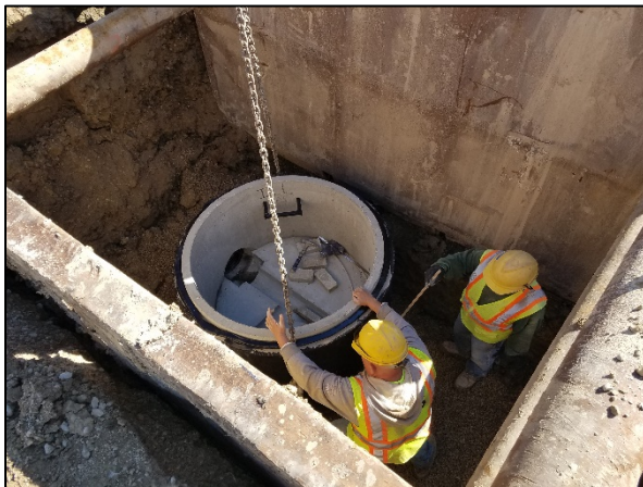
Lake County Grading setting the base for a manhole.
