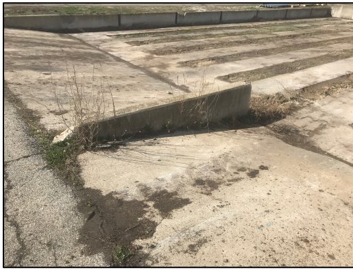
Concrete dividing wall in apron
