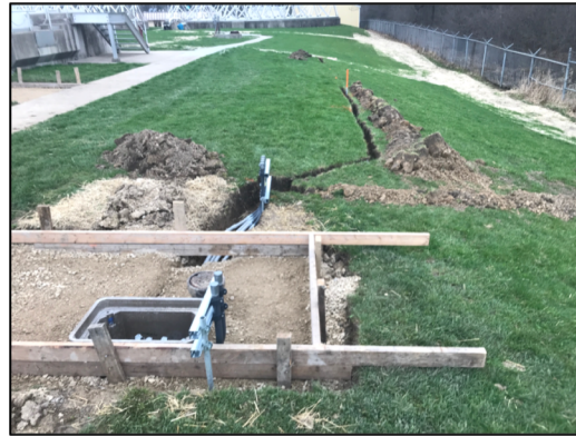
Conduit & junction box installed at future control panel site.
