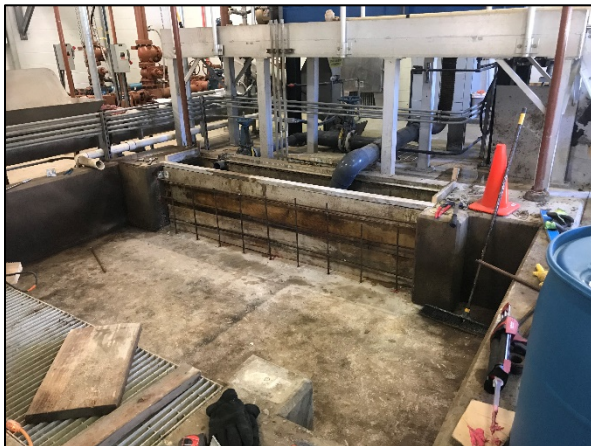
Picture of rebar in place for new concrete divider.
