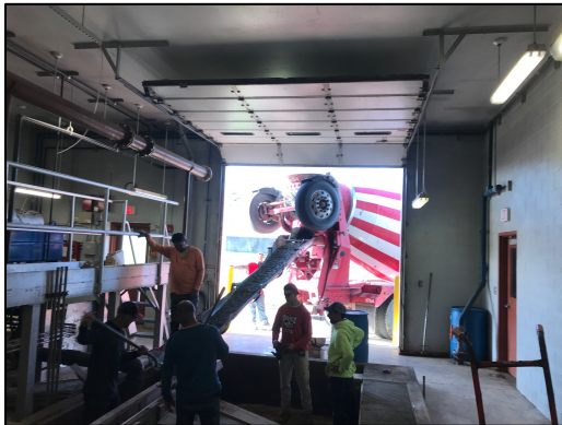
Concrete for dividing wall being poured.
