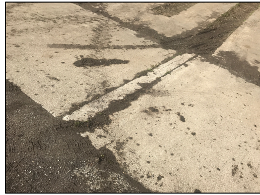
Dividing wall removed.
