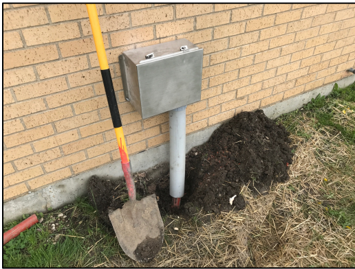
One of several junction boxes that were installed.
