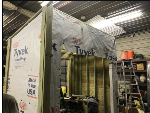
Dumpster Enclosure with roof and moisture barrier.
