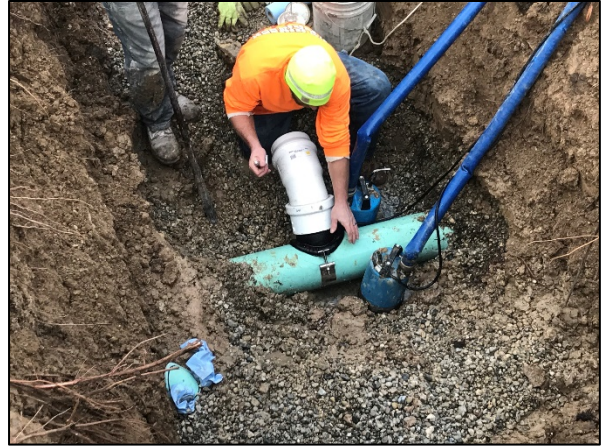
Picture of crew attaching the service line.
