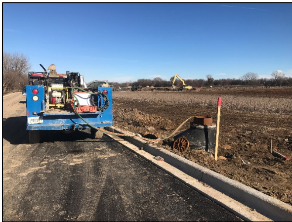
Picture of the testing apparatus used for the sanitary air tests.
